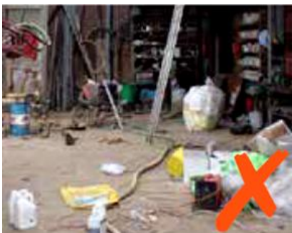
Mess creates risk
