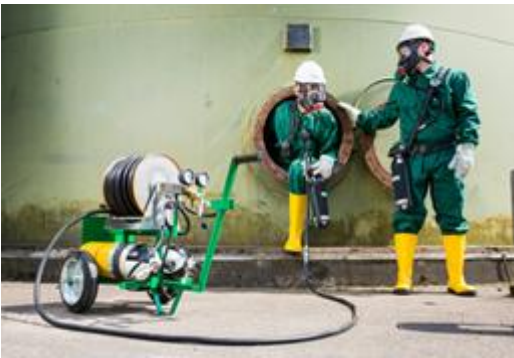
Organised work in a confined space
